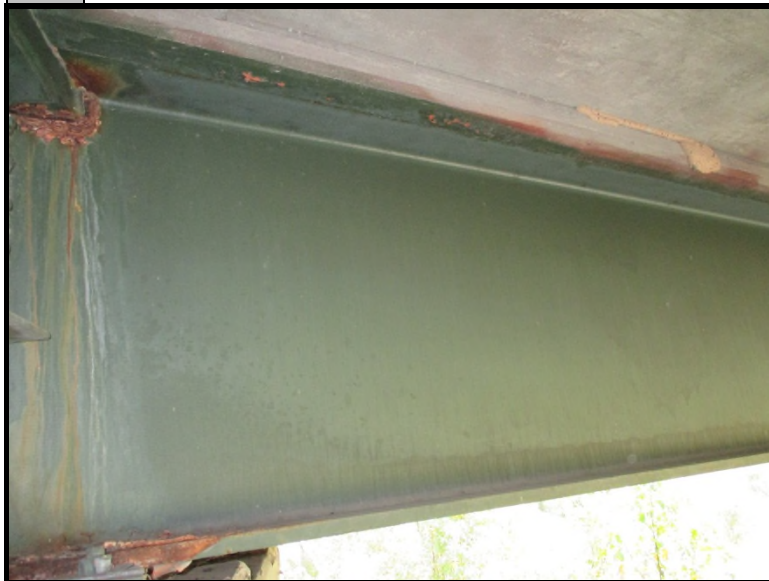
3 The green painted I-beams, bolt plates and braces tested positive for lead-based paint.
