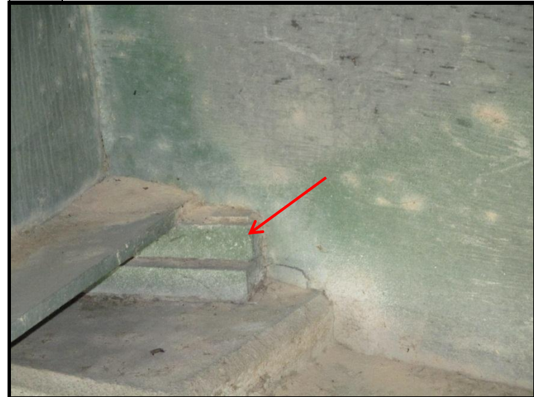
4 The green paint on the bolt plate tested positive for lead-based paint (1.4-2.6 mg/cm 2 ).
