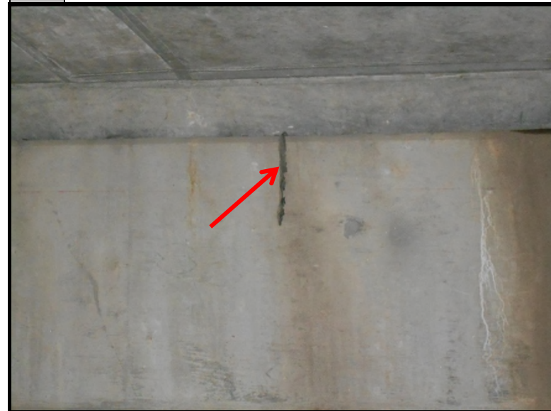
4 The tar paper associated with the bridge tested negative for asbestos.
